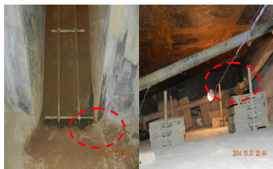
图9 浆液从加荷板底部及斜坡面下部同时冒出 Fig.9 Slurry flow out from the bottom plate and slope bottom
